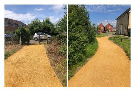
**Footpaths exiting onto Dozule Close.** The final part of these paths have been surfaced by Gloucestershire County Council (LSPC paid for them to be finished with top stone), the vegetation has been cleared and the hoop from the Kissing Gate removed making it a simple pedestrian gate, vastly improving the access and safety.
